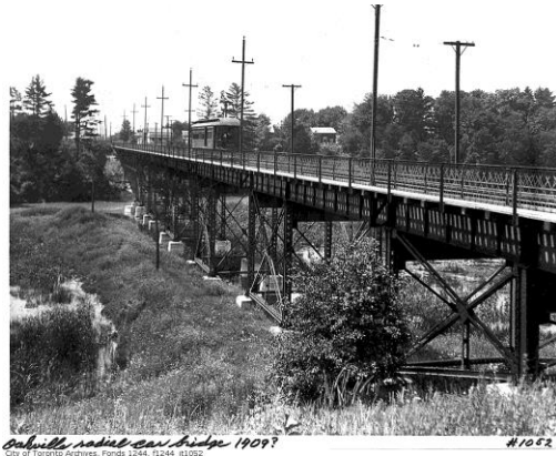
Oakville radial car bridge 1909?
