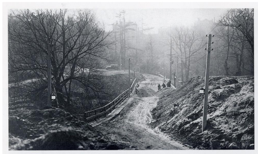
Photograph-Roxborough Street E. near Mount Pleasant Rd. 1927 Dept. of Public Works Tor. Ref. Library 976-47-6
