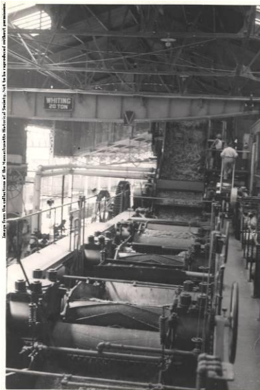
Interior view of machinery at the Soledad sugar mill, near Cienfuegos, circa 1930 – 1940, from the Atkins family photographs, Massachusetts Historical Society. Soledad Mill, Atkins Family Photographs
