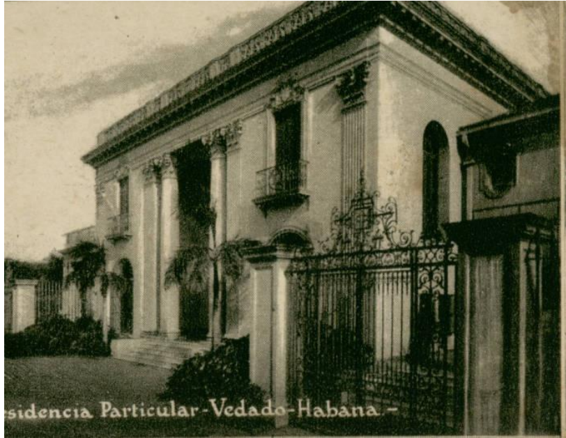
Cuba en 1925, Susini El Cigarro Sin Rival Album for souvenir pictures enclosed in tobacco products. Images of politicians, buildings, and places of interest of the six Cuban provinces in 1925. detail p. 23. Hastings-designed residence
