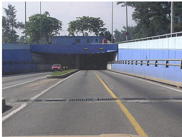
Panoramio Roberto Lam Tunnel to Miramar
