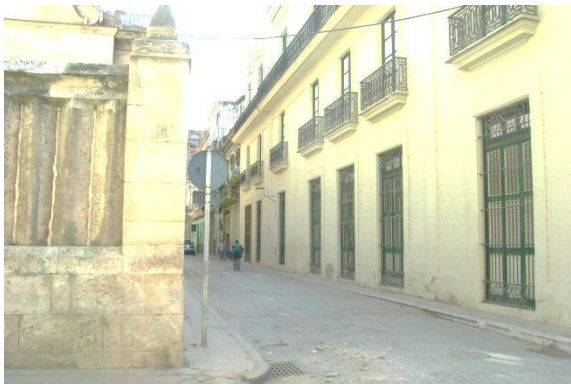
Aguiar facade (photo T. Casas 2009)
