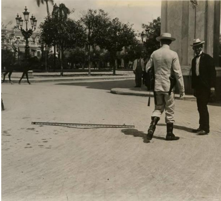
testing the pavement
