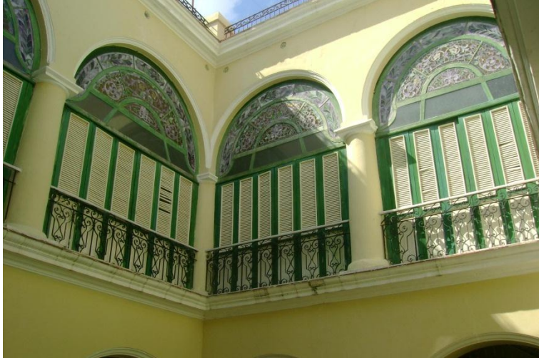
“Two wide galleries with wooden shutter-blinds (persianas) and semi-circular stained glass transept windows (medio puntos de cristales.)”
